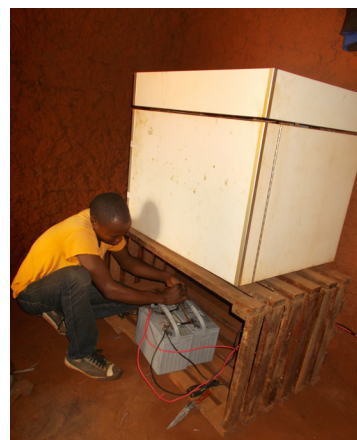
A technician repairs a solar refrigerator in Congo.
